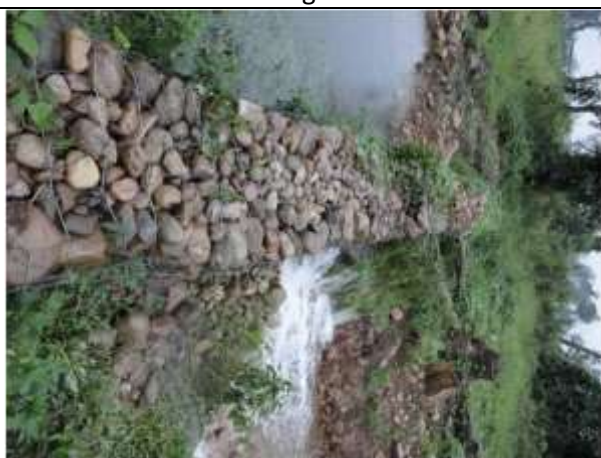
Filtered check constructed across natural drain CHF, Pasighat
