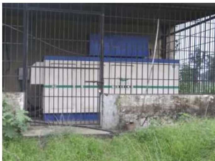
200KVA DG Set for uninterrupted power supply
